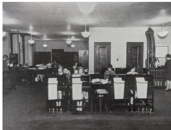
Figure 22: The acoustic treatment in a women working space: Absorbent felt on the ceiling and pneumatic tube also acoustically treated
